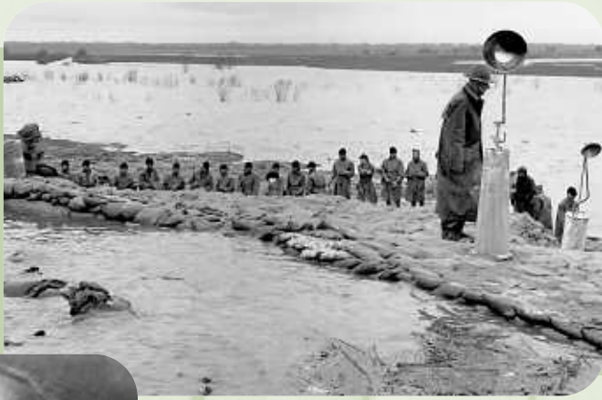
Sandbagging a levee during flooding of the Mississippi River
