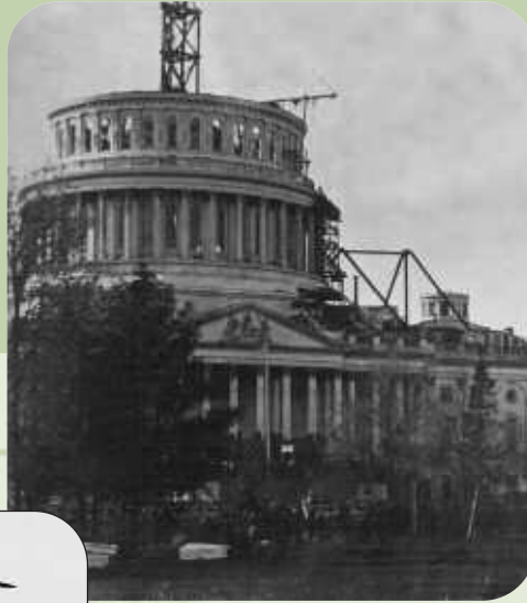
Capitol dome under construction, 1861
