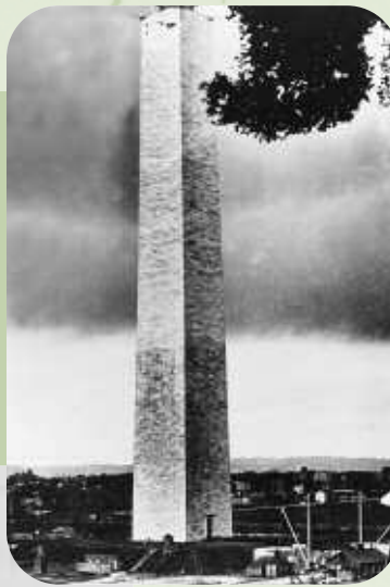
Washington Monument nearing completion, early 1884 National Archives
