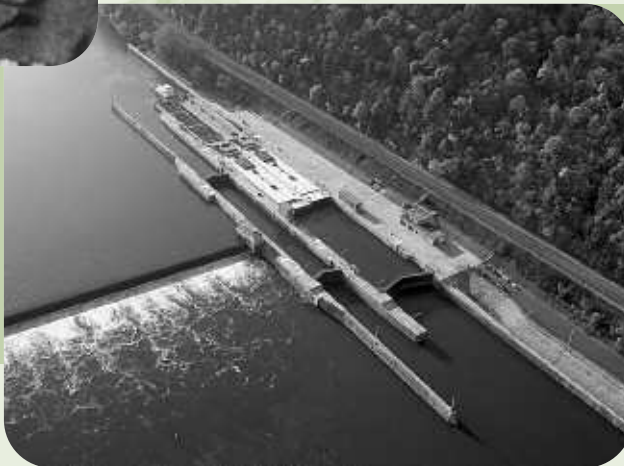
Dashields Locks and Dam on the Ohio River near Glenwillard, Pa., opened for navigation August 1929.
