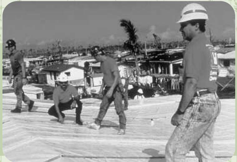
Installing temporary roofs following Hurricane Andrew
