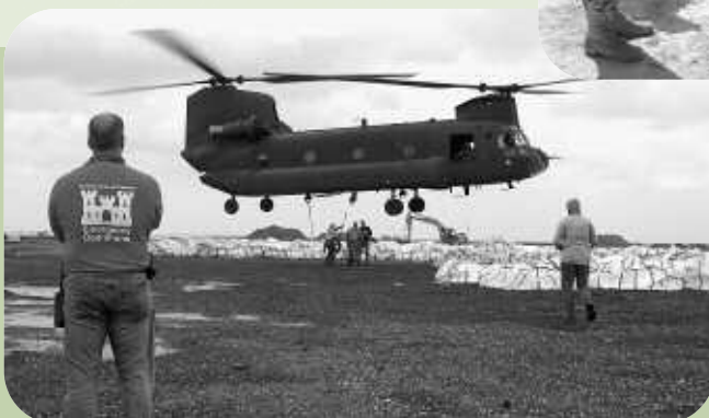
Chinook helicopter prepares to lift 5,000-pound sandbags to repair damaged flood walls.
