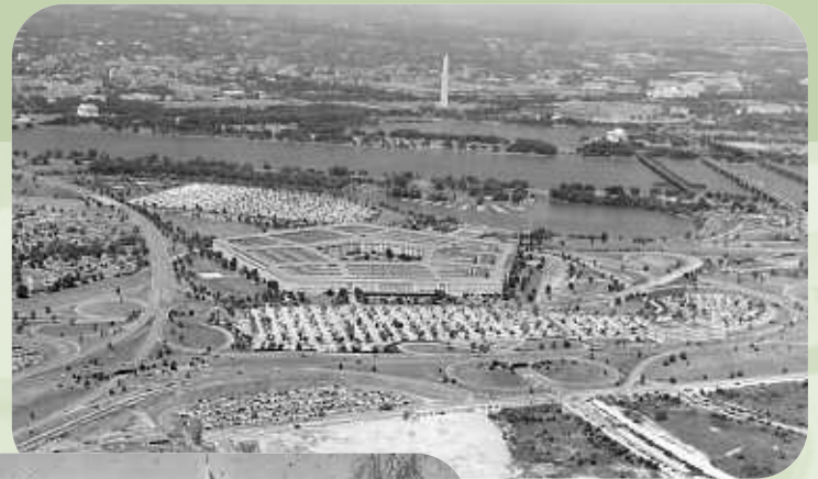
An aerial view of the completed Pentagon
