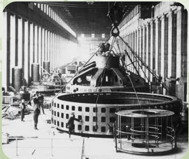
The power generators at Wilson Dam, Tenn., under construction, 1926
